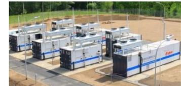
Water electrolyser units to generate H<sub>2</sub> for injection into existing regional natural gas transmission system
